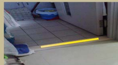
A bright yellow "anti-slip tape" can highlight the threshold to avoid trips.
